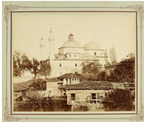
Figure 2 General view of the Green Mosque
